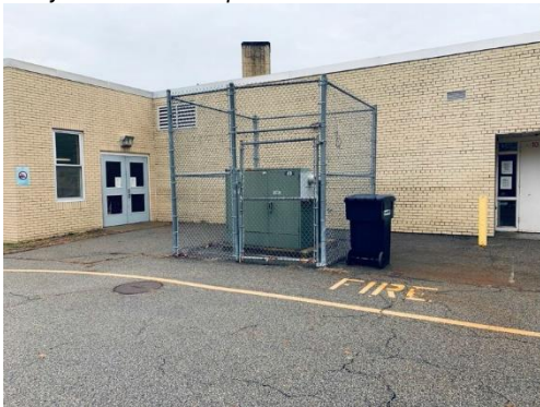
Utility Co. Pad-mount Transformer
