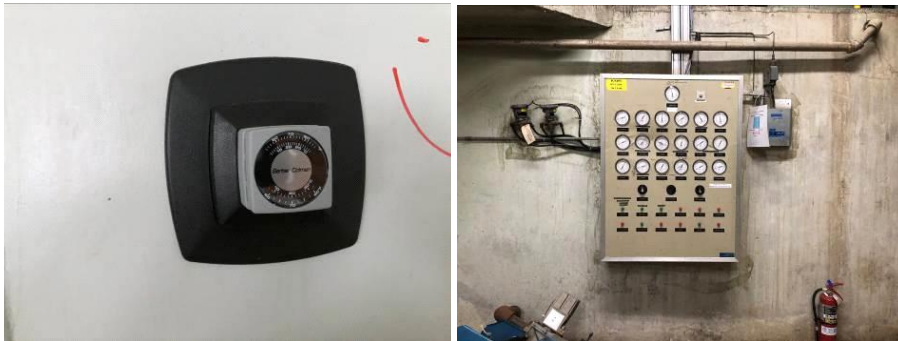
(L - Pneumatic Thermostat, R - Pneumatic Control Panel)
