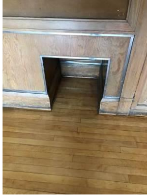
(L - Typical Classroom Exhaust Opening, R - Roof Exhaust Fans)
