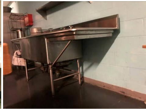
(L - Wall-hung Urinals, R - 2-compartment pot sink without interior grease trap)
