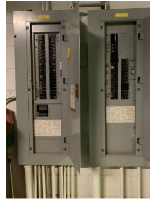
Feeder Circuit Breakers Panels
