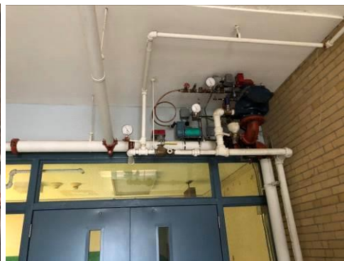
(L - Sprinkler Riser Station, R - Dry Sprinkler Valve)
