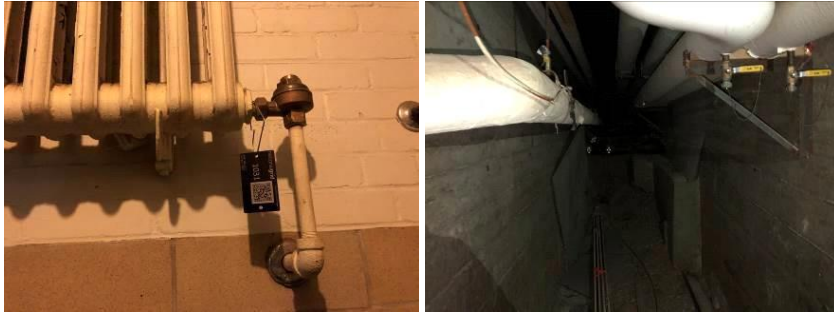
(L - Steam Radiator and Steam Trap, R - Steam Pipe Tunnel)
