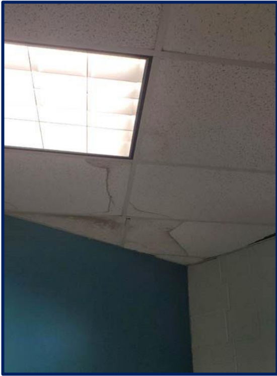
Photograph #9 – Water Damage in Library – 1988 Addition
