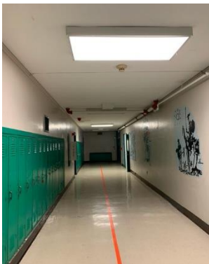
Corridor surface 4'x4' – 4 lamp fluorescent light fixtures
