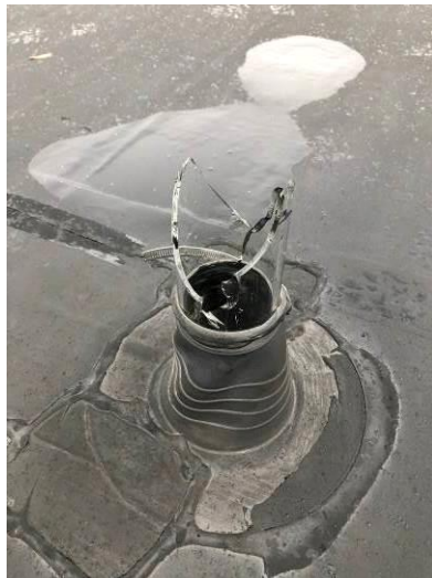
(L - Roof Leak at Damaged Glass Acid VTR, R - Emergency Eyewash/Shower Station)
