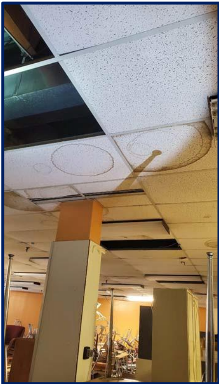
Photograph #10 – Water Damage in “Cafeteria” (1) – 1988 Addition
