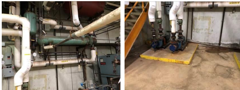
(L - Steam-to-Hot Water Heat Exchanger, R - Hot Water Pumps)
