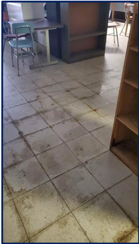
Photograph #11 – Water Damage in “Cafeteria” (2) – 1988 Addition
