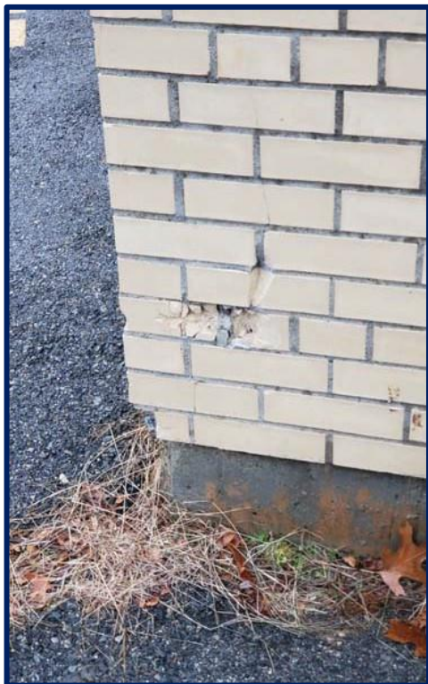
Photograph #11 – Water Damage in “Cafeteria” (2) – 1988 Addition
