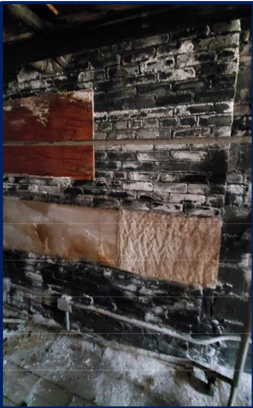
Photograph #6 – Efflorescence Masonry Wall in Loft Area – 1952 Addition
