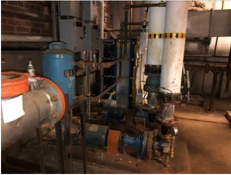
Hot Water Pumps P-1 and P-2
