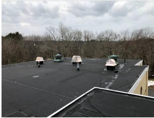
(L - Typical Classroom Exhaust Opening, R - Roof Exhaust Fans)
