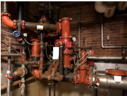
(L - Sprinkler Riser Station, R - Dry Sprinkler Valve)
