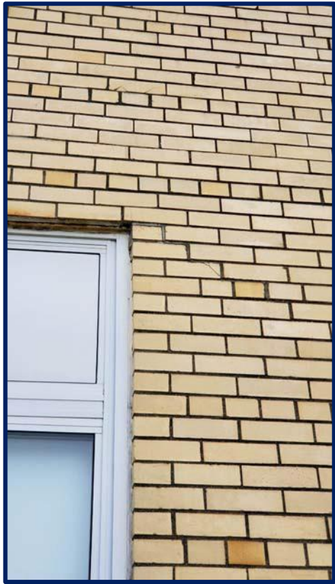
Photograph #13 – Cracking Caused by Corroded Lintels – Multiple Locations
