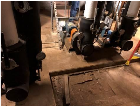
(L - Air-Cooled Chiller, R - Triplex Chilled Water Pumps)
