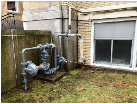
(L - Gas Service and Gas Meter, R - Horizontal Domestic HW Storage Tank)
