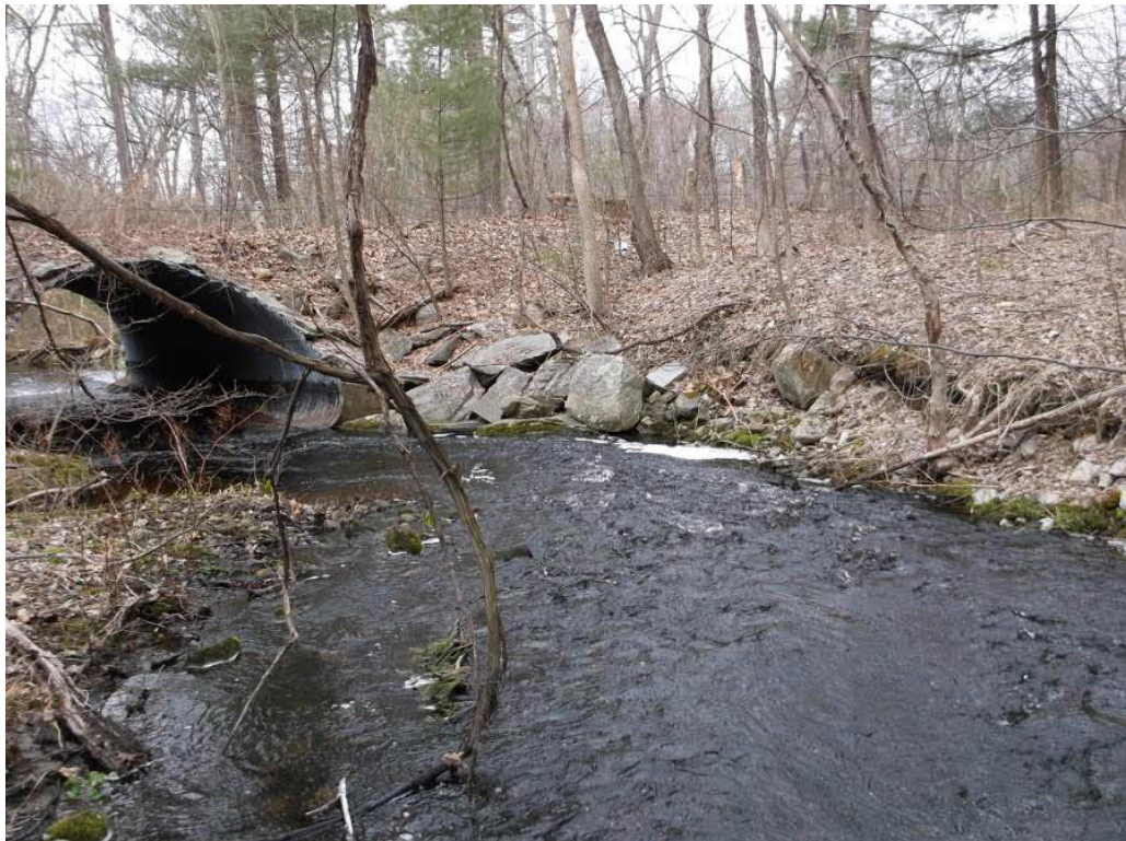
Photo 6: Northeast embankment erosion.
