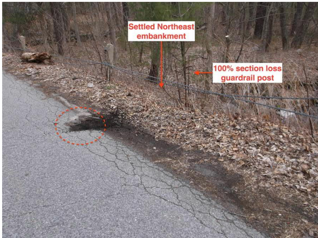
Photo 5: Wearing surface and North approach pavement, looking Northeast. Settlement in Northbound lane is circled. East rail post with 100% concrete section loss indicated (only rebar remaining).
