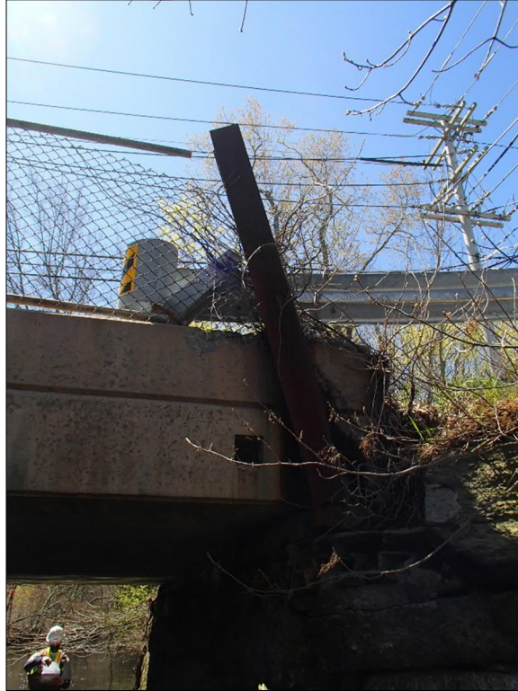
Photo 21 Looking Southwest: Post Damage at North Approach Guardrail
