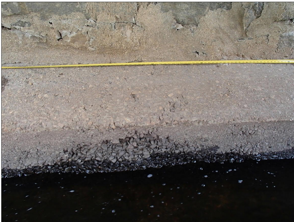
Photo 10 Looking West: Scaling and Abrasion at Concrete Apron
