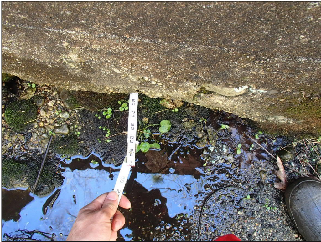
Photo 7 Looking South: Southwest Wingwall Void
