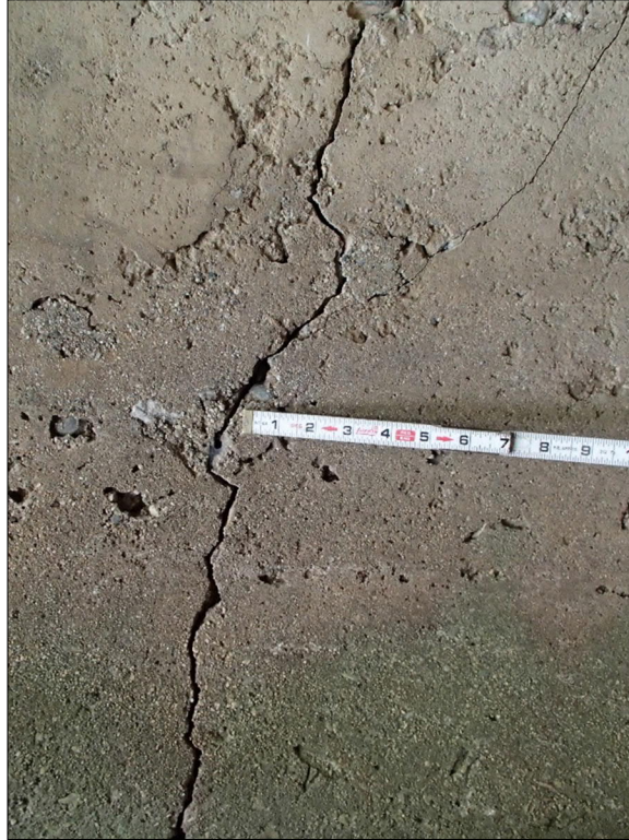
Photo 9 Looking North: Crack near West End of North Abutment
