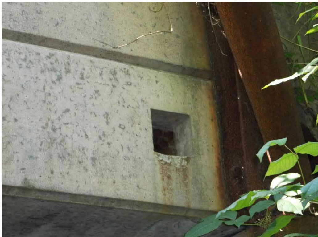
Photo 6: Northwest post-tensioning hole, typical rusted assembly.
