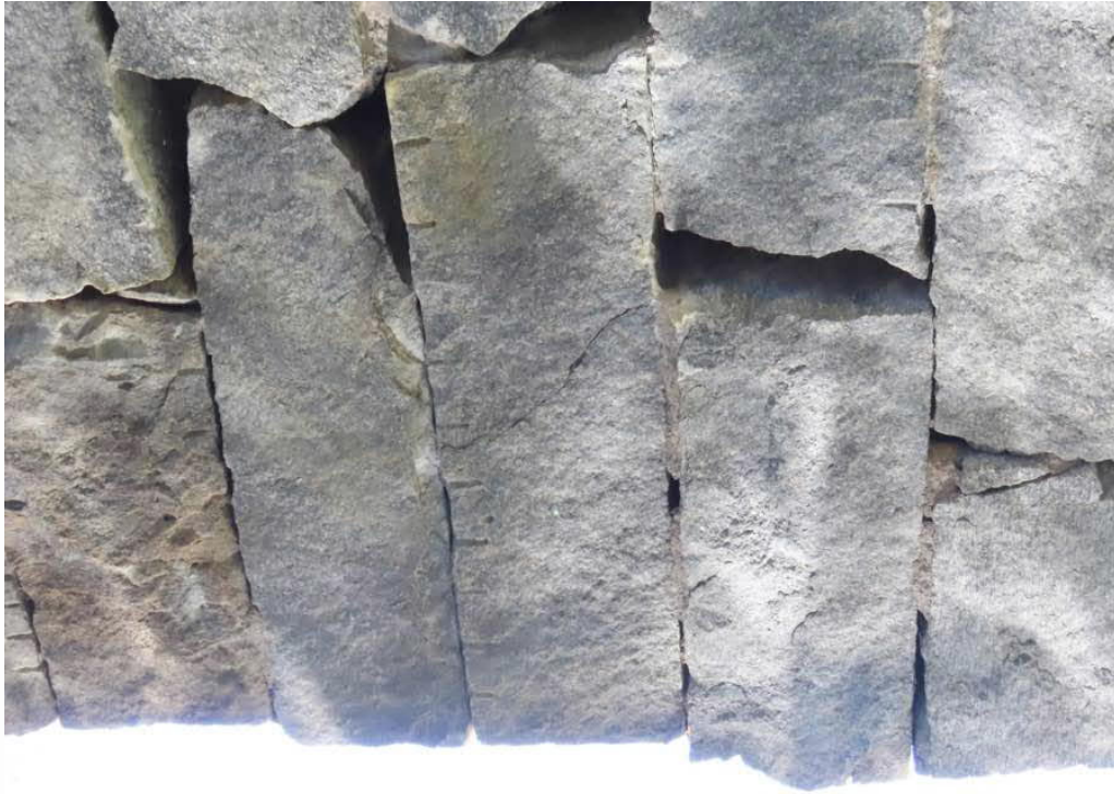
Photo 7: Cracked South archring stone near the keystone.
