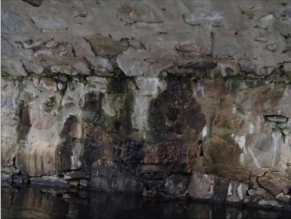
Photo 11 Looking South: South Abutment Water Stains
