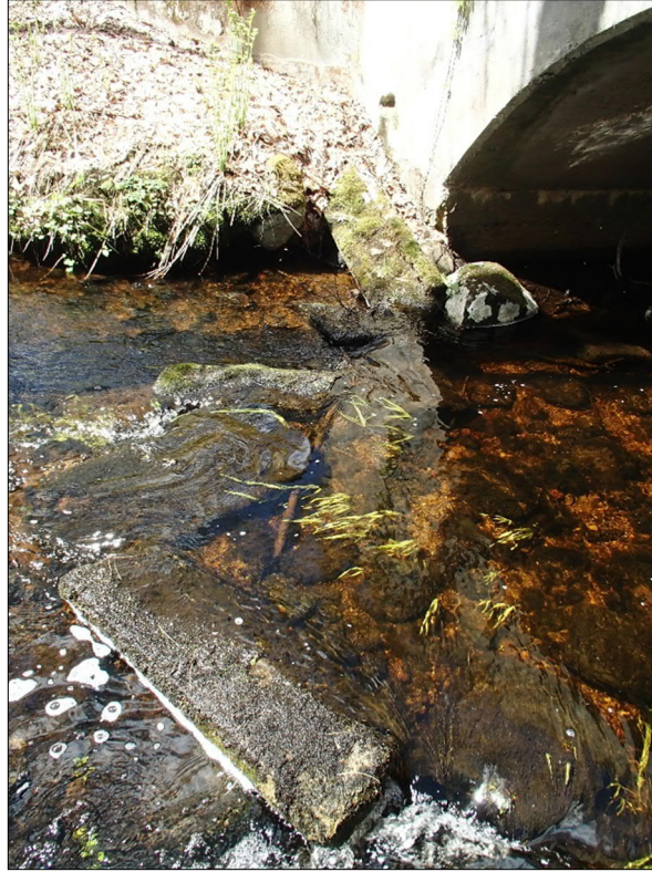
Photo 9 Looking South: Debris at East Entrance to Culvert
