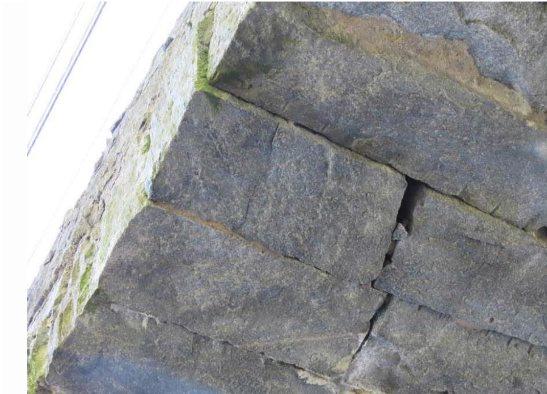
Photo 9: Cracked North archring stone West of keystone.
