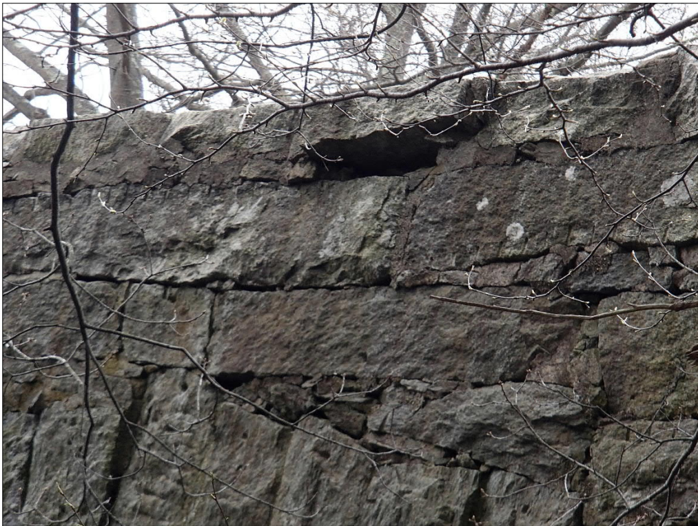
Photo 10 Looking South: North Coping Stone Movement
