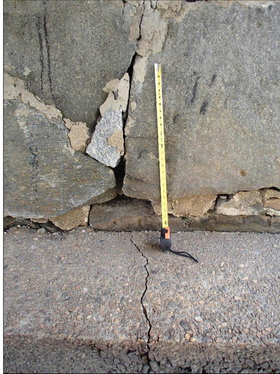
Photo 11 Looking West: West Abutment Voids and Apron Cracking
