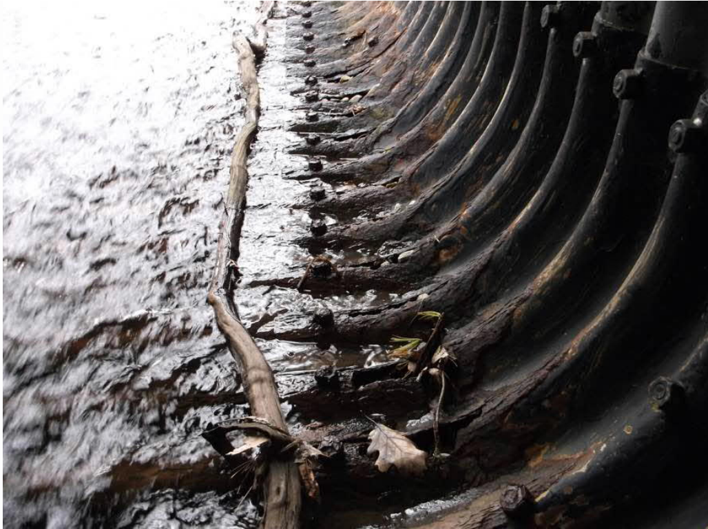
Photo 1: South waterline looking East, typical 100% section loss.
