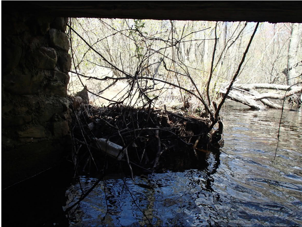
Photo 13 Looking North: Vegetation Impeding Flow at Northwest Corner
