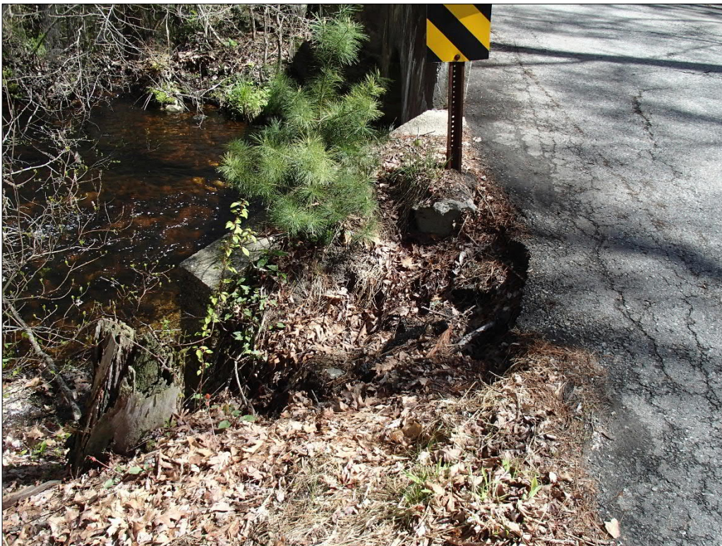
Photo 14 Looking North: Collapse behind Southwest Wingwall
