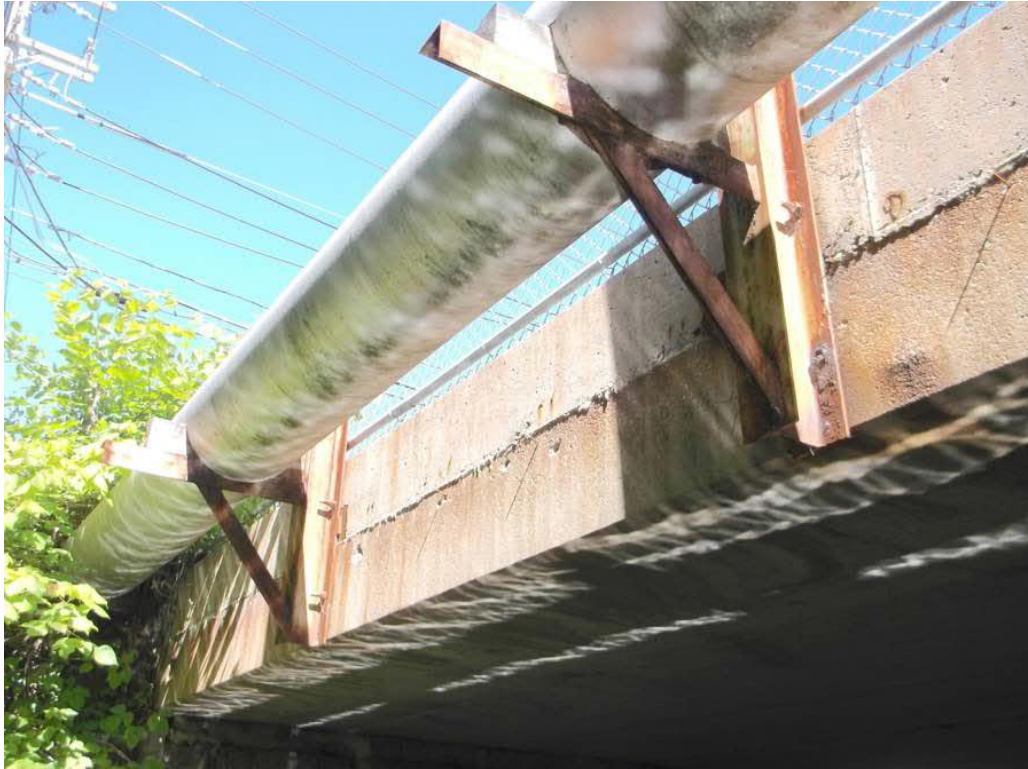
Photo 3: South fascia, rusted utility supports.
