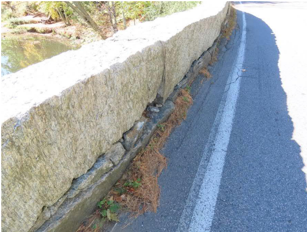
Photo 2: Minor misalignment of the parapet stones. South parapet.
