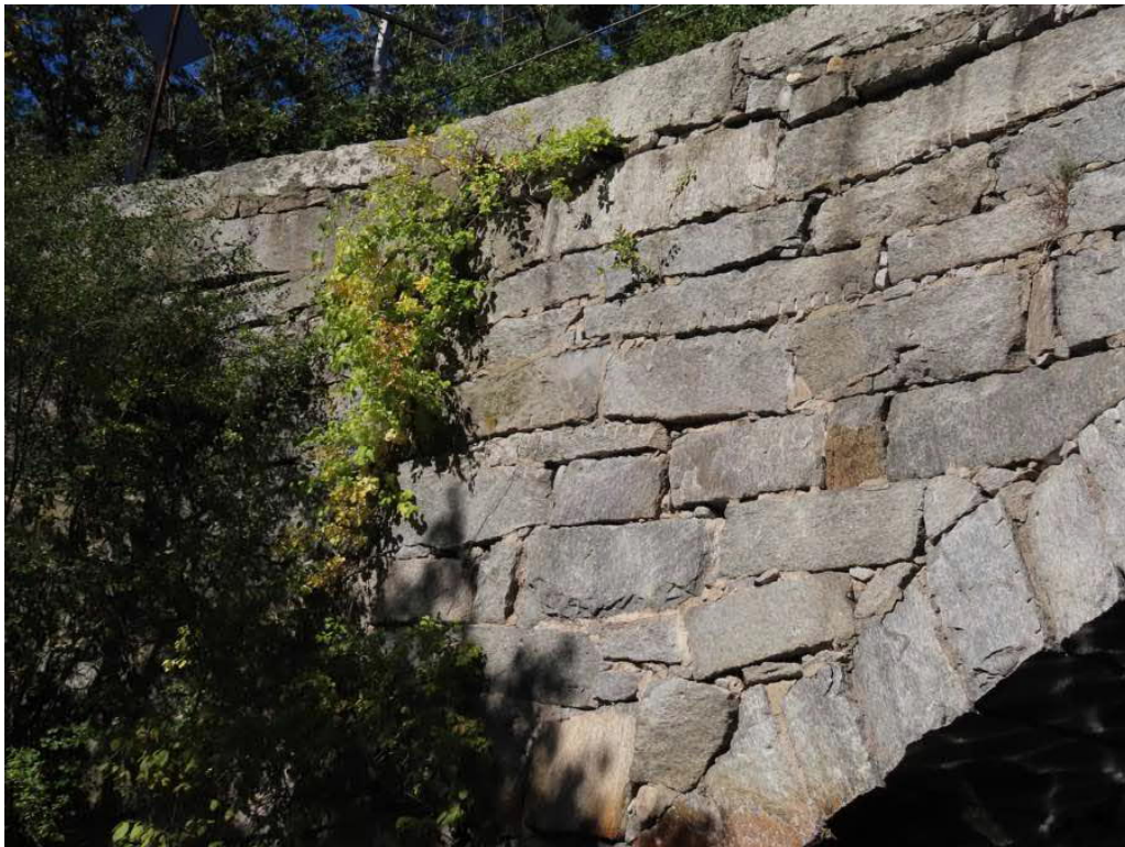
Photo 10: Vegetation growth at the West end of the South spandrel wall.
