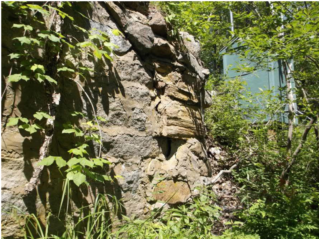
Photo 10: Northeast wingwall displacement, looking North (from channel).
