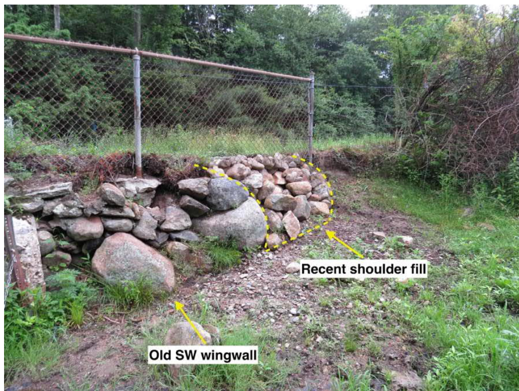
Photo 4: Southwest wingwall and shoulder fill.
