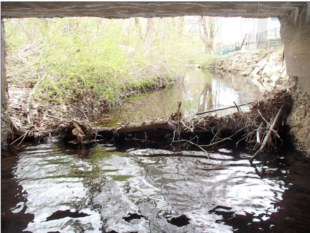
Photo 20 Looking West: Debris at West Entrance
