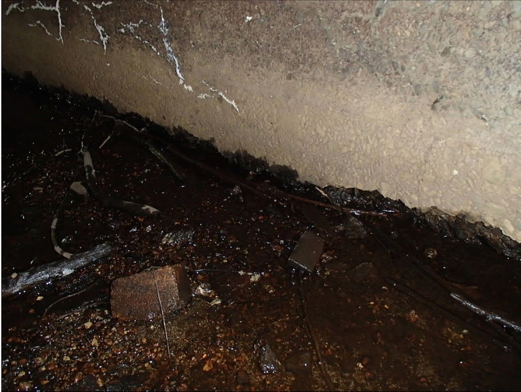
Photo 19 Looking North: Abrasion at Water Line
