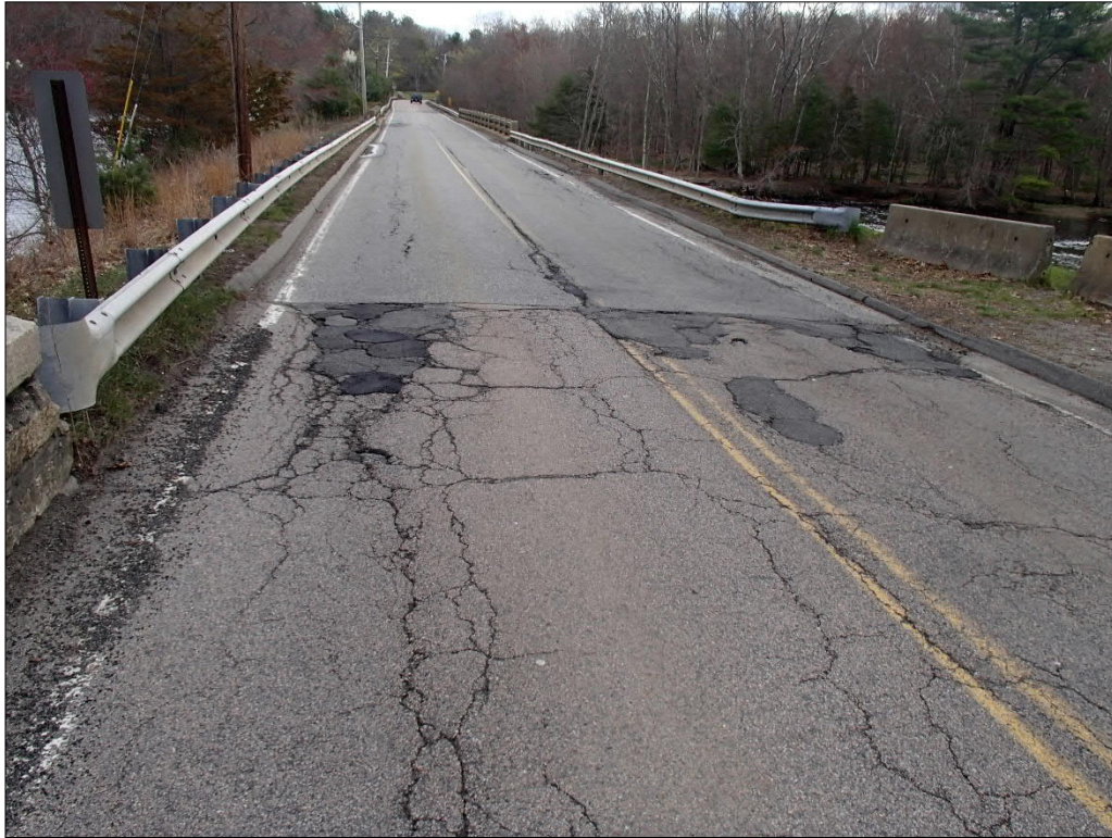
Photo 13 Looking East: Patching Near East Approach
