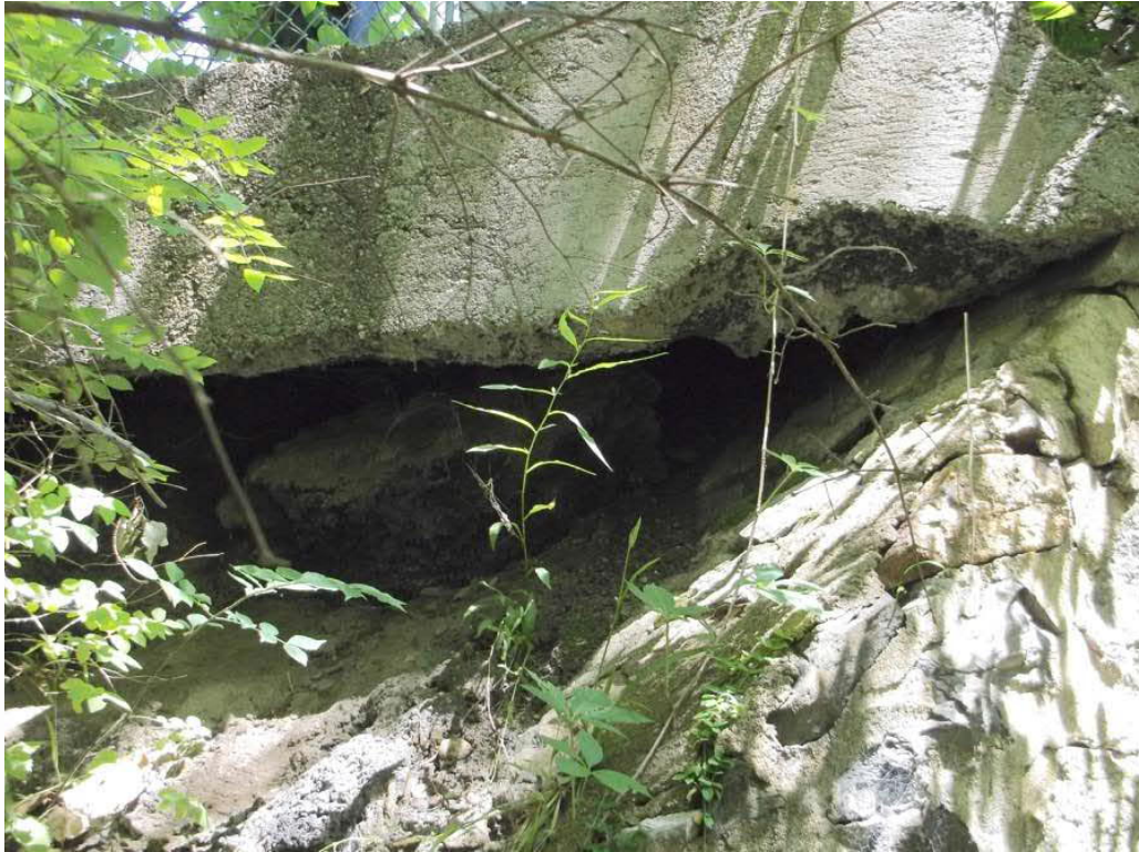
Photo 11: Northwest wingwall cap void (note bituminous chunk).
