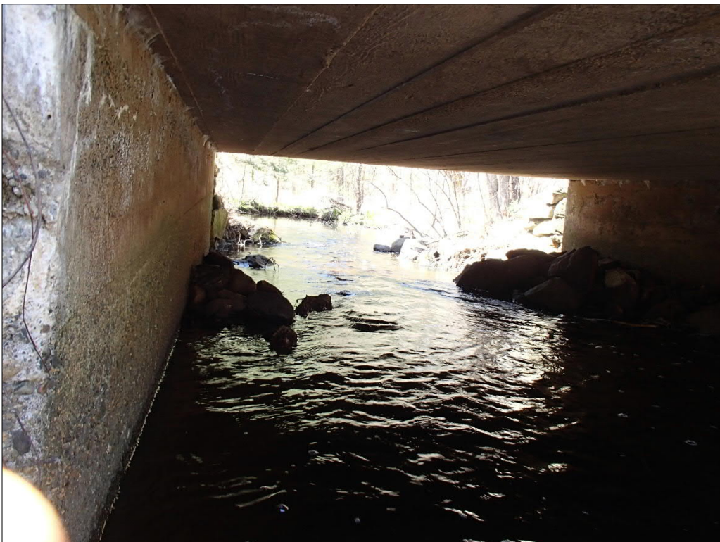
Photo 10 Looking South: Debris Under Culvert
