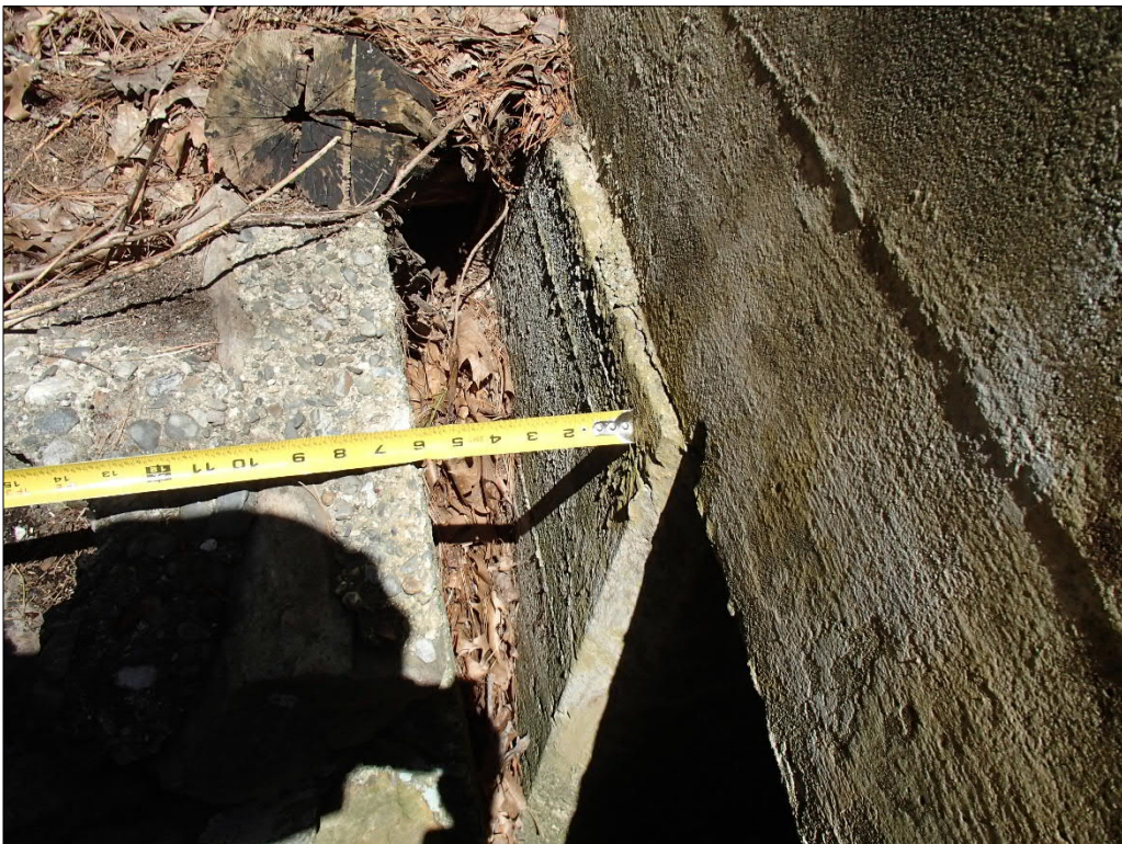
Photo 14 Looking North: Separation of Northwest Training Wall and Culvert
