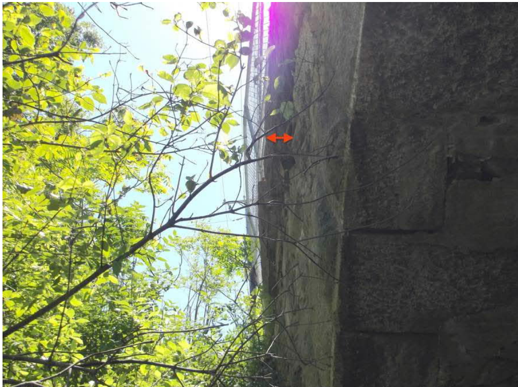
Photo 8: East spandrel wall South end, looking South, capstone displacement.
