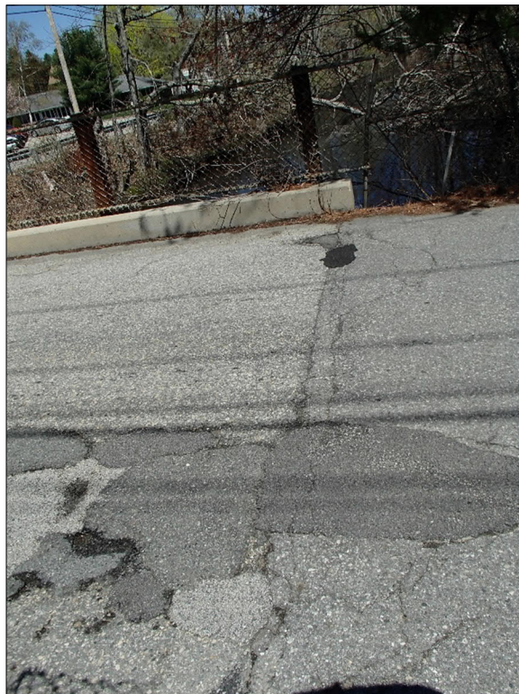
Photo 22 Looking North: Cracking at East Joint
