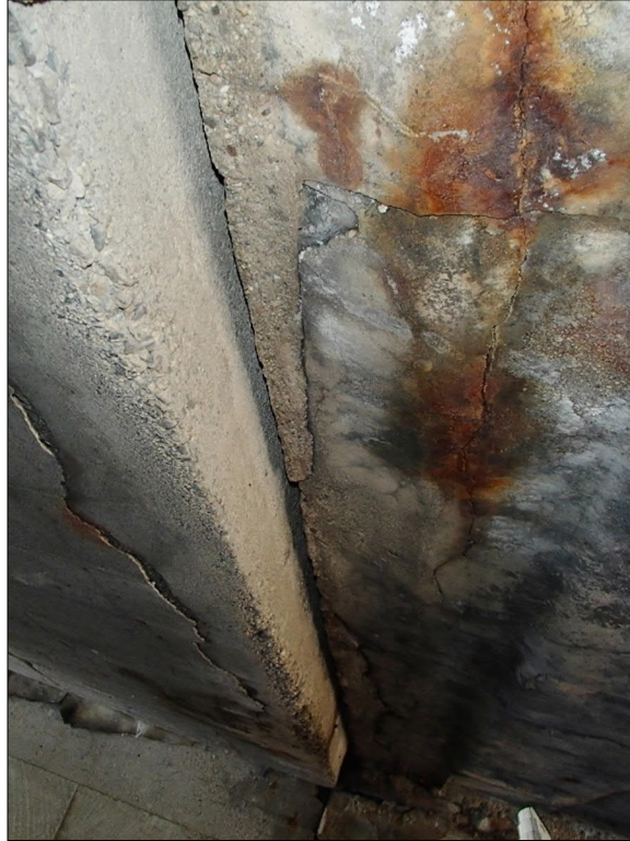
Photo 7 Looking West: Culvert Roof Interface – Shows Cracks w/ Rust Stains & Efflo.
