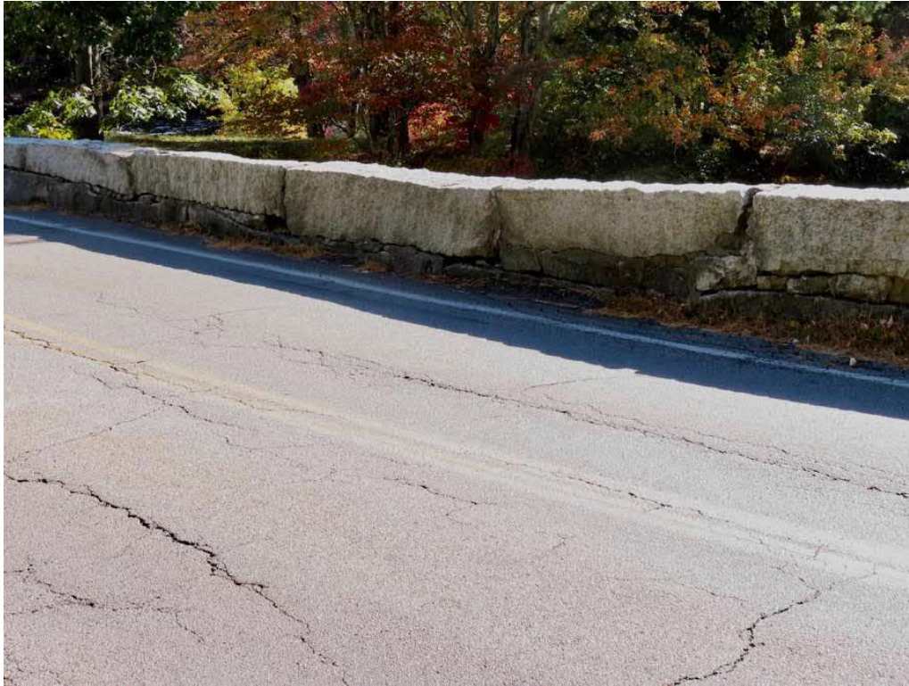
Photo 1: Cracking to the wearing surface.
