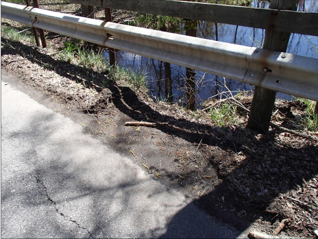
Photo 21 Looking South: Washout at Southwest Corner over Culvert
