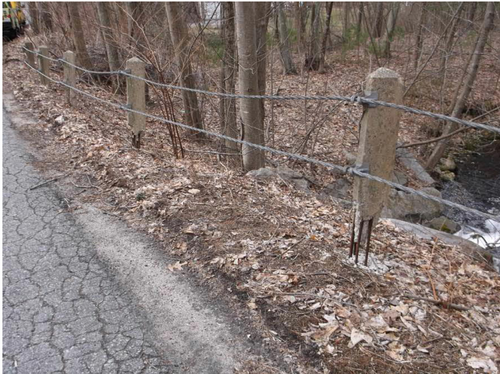
Photo 7: West rail South end, typical post concrete section loss.
