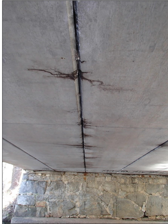
Photo 9 Looking East: Cracking and Staining at Beam Joints
