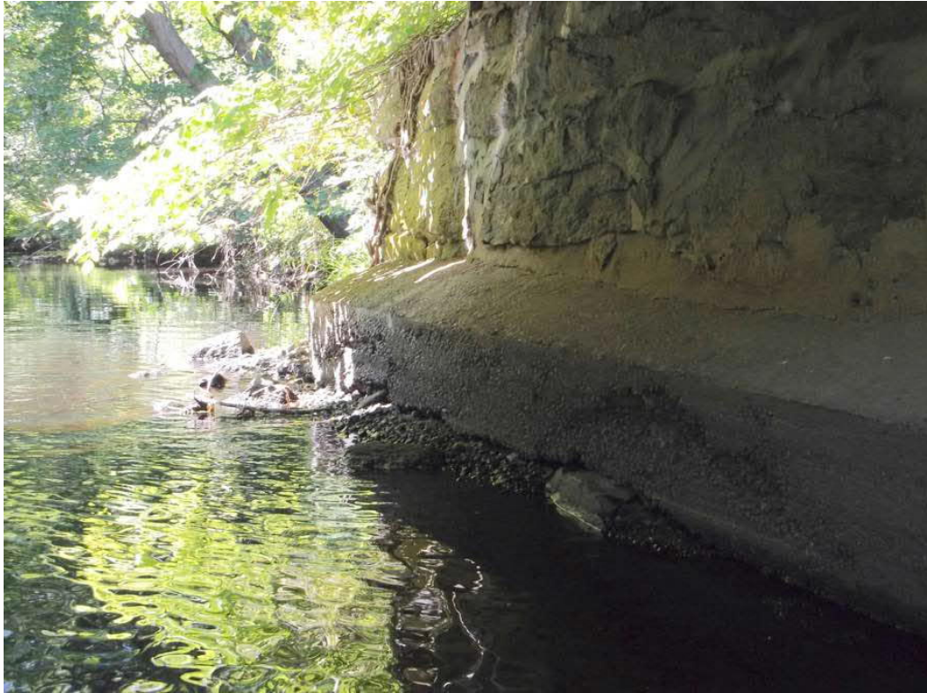
Photo 7: West concrete apron looking Southwest, abrasion and undermining.
