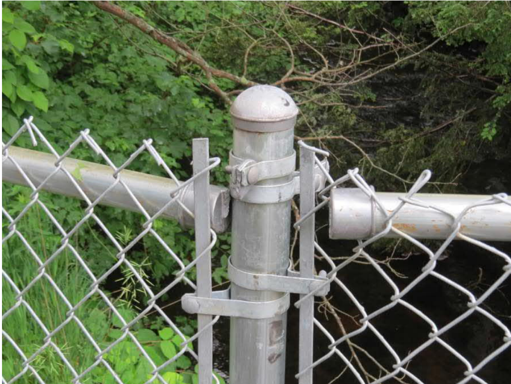
Photo 3: East fence North end, disconnected top rail.
