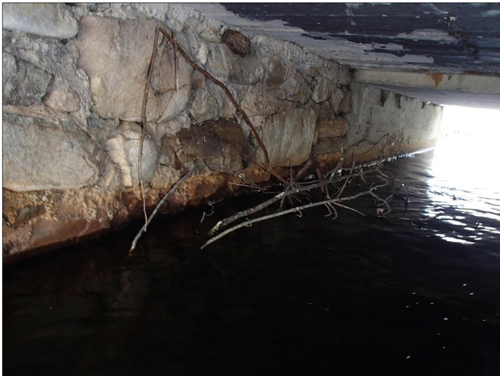
Photo 14 Looking Southeast: Debris in Brook at East Abutment Wall
