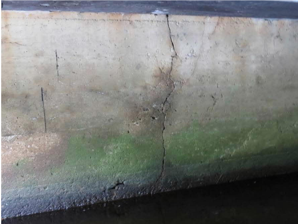
Photo 7: North breastwall settlement crack, 6' in from West end.
