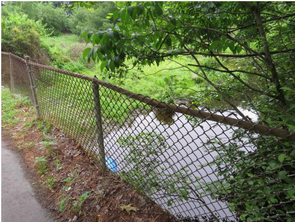
Photo 2: West fence, bent top rail.
