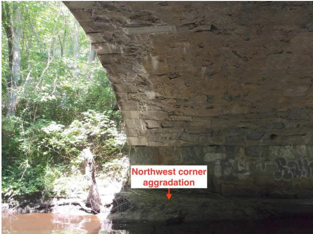
Photo 7: West side, looking North, concrete cover deterioration and aggradation.
