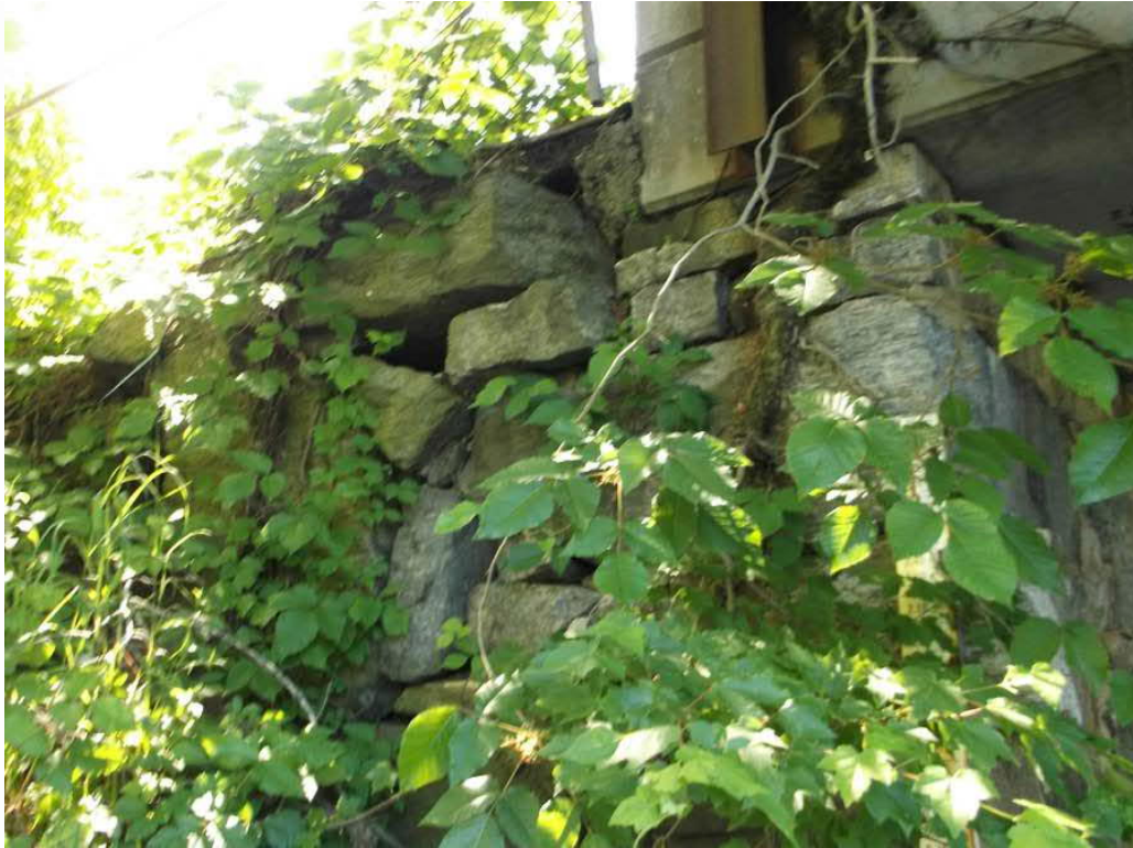
Photo 9: Northeast wingwall, voids and displaced stones.
