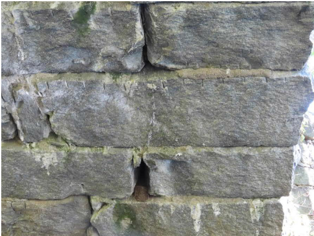
Photo 8: Cracked South archring stone above East breastwall.
