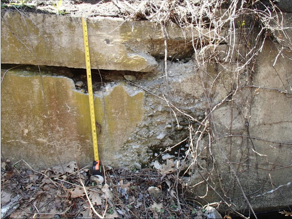
Photo 13 Looking East: Cracking and Spalling of Southeast Wingwall
