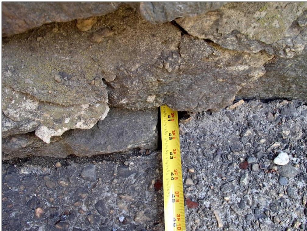
Photo 12 Looking East: Void at East Abutment
