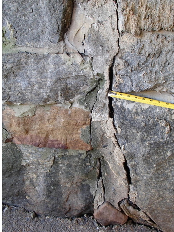
Photo 13 Looking East: Full Height Crack at East Abutment
