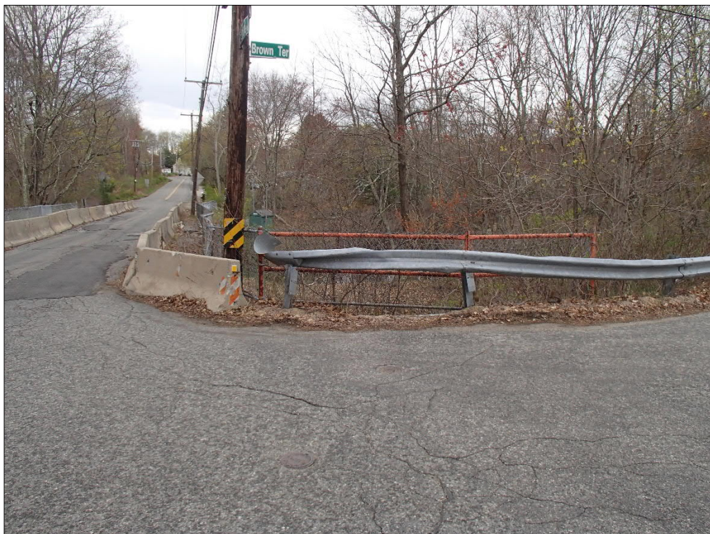
Photo 18 Looking North: Collision Damage on Southeast Approach Guardrail
