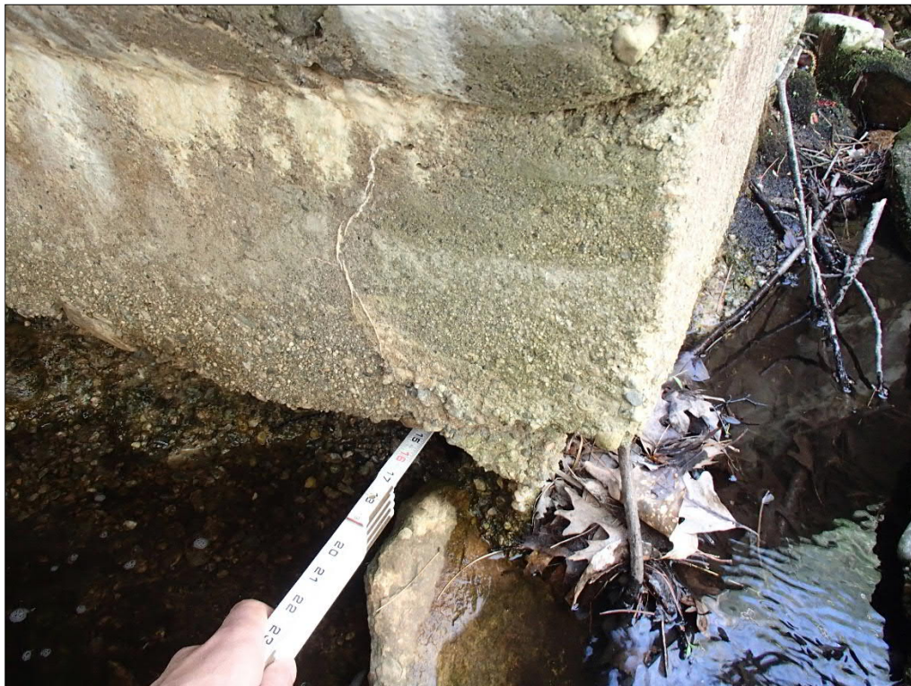
Photo 8 Looking South: Southwest Abutment Corner Void
