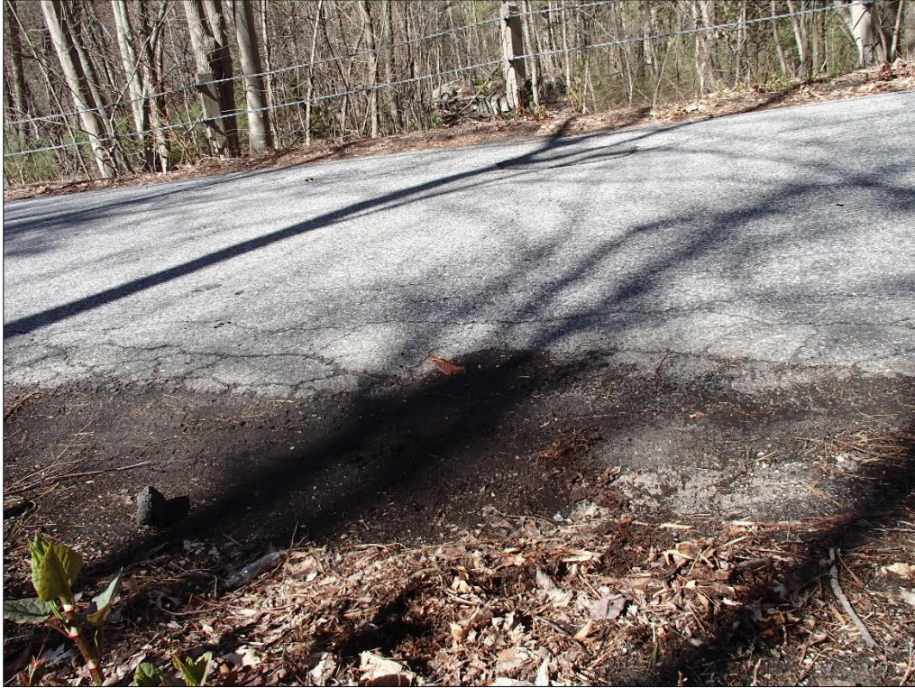
Photo 19 Looking West: Washout/Settling near Northeast Corner over Culvert
