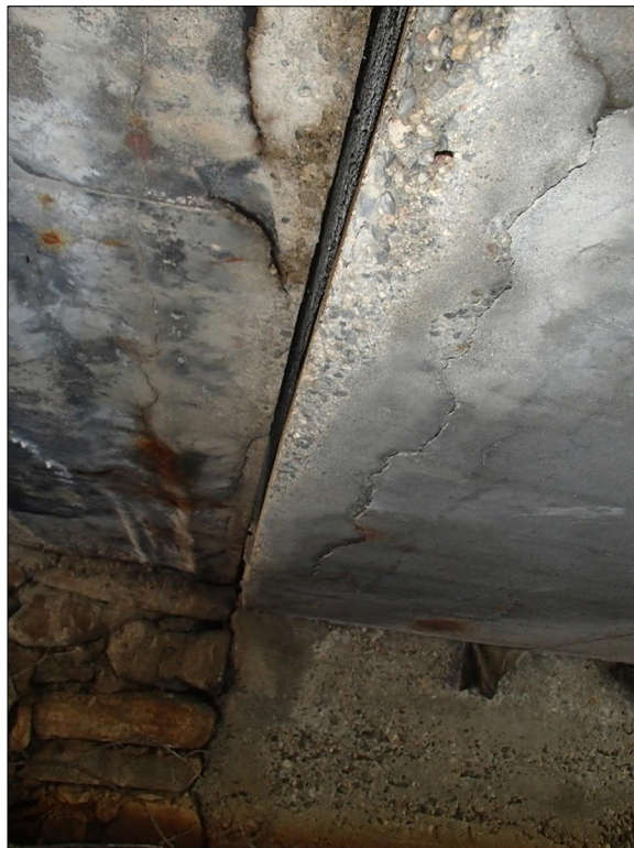
Photo 8 Looking East: Culvert Roof Interface – Shows Cracks w/ Rust Stains & Efflo.
