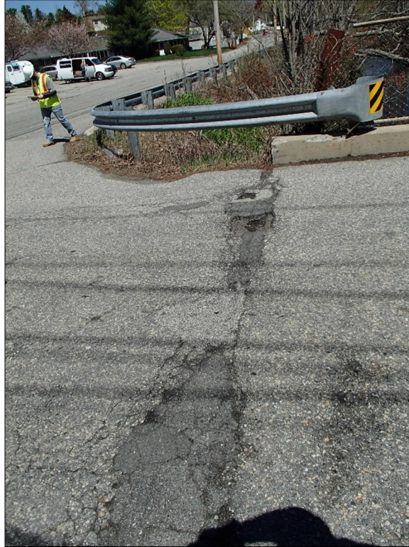
Photo 23 Looking North: Cracking at West Joint
