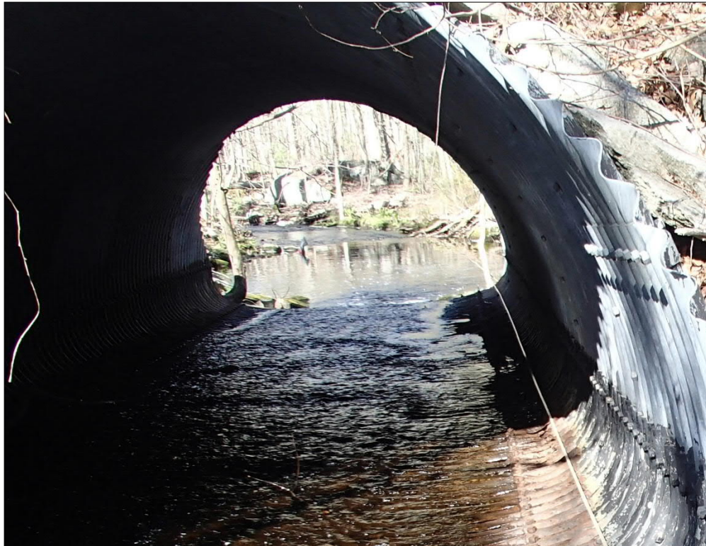
Photo 14 Looking West: Distortion of Pipe
