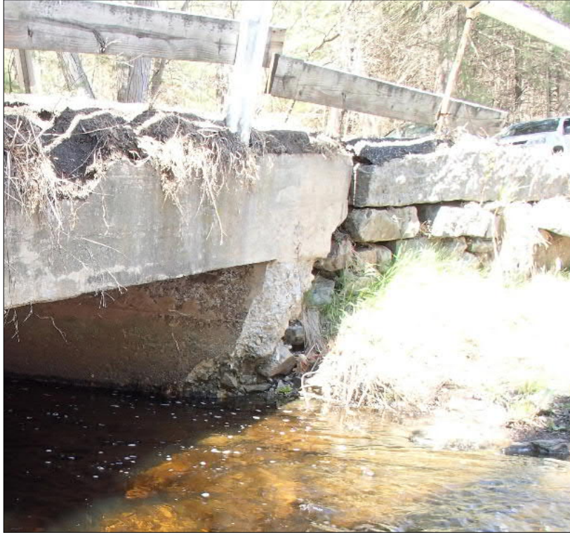
Photo 11 Looking Northwest: Spalling at Northeast Abutment Corner
