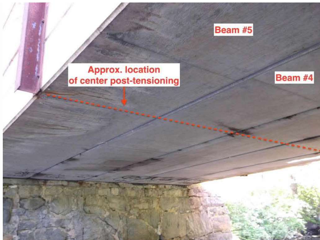
Photo 5: Underside of beams looking Southeast, typical moisture stains.
