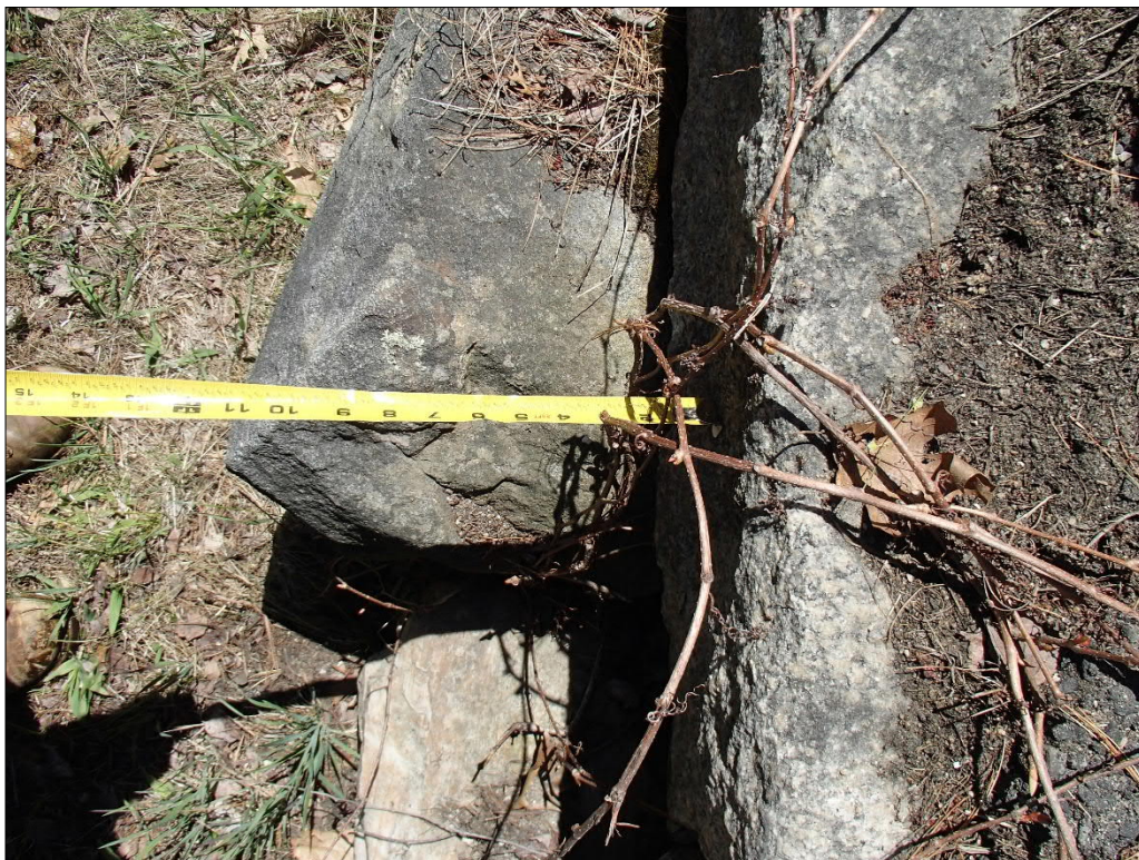
Photo 12 Lateral Displacement of Northeast Wingwall
