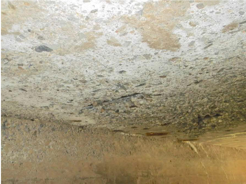
Photo 3: Span #1 center, poor consolidation.
