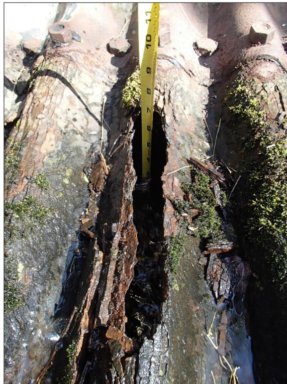
Photo 8 Looking North: Section Loss at North Wall of Pipe
