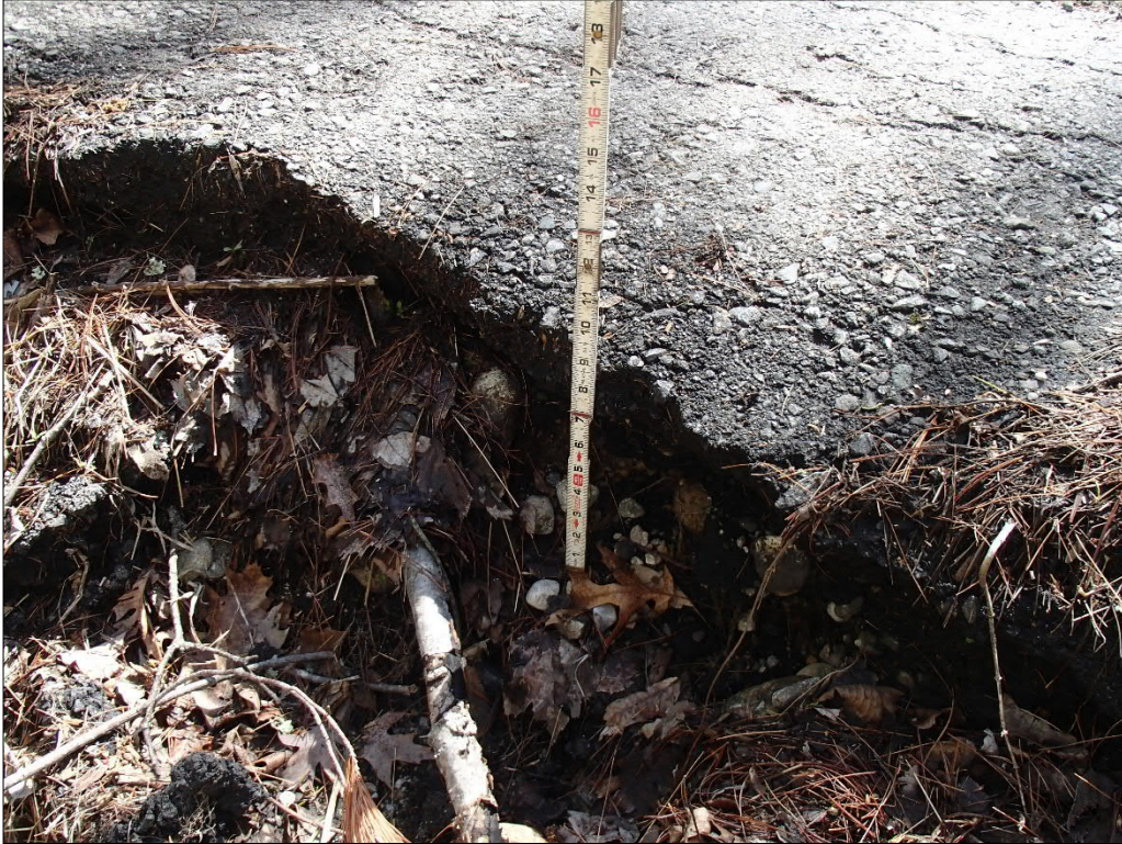
Photo 15 Looking East: Undermining of Pavement near Southwest Wingwall
