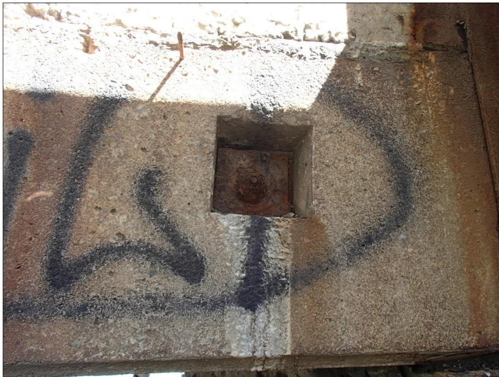
Photo 14 Typical Corrosion of Post Tension Ties
