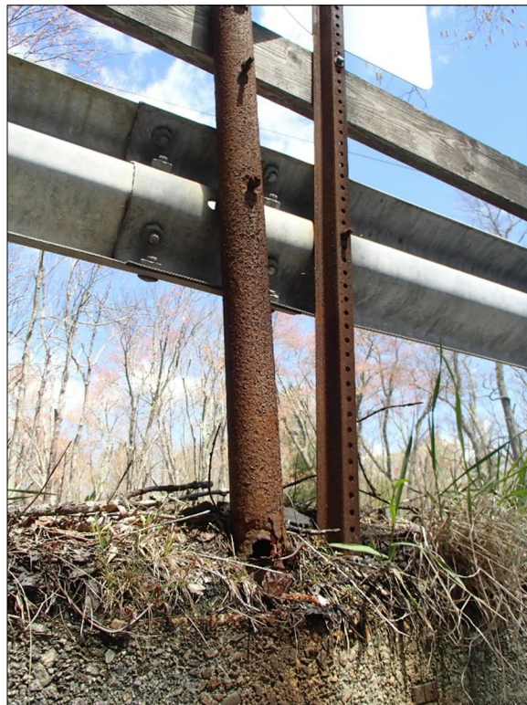
Photo 22 Looking North: Rust at South Railing
